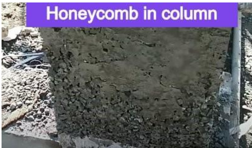
Fig 2: Honeycomb in Column
