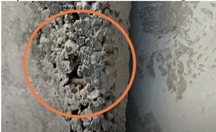
Fig 1: Honeycomb in Wall
